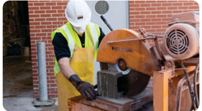
Cutting concrete block with water
