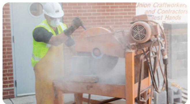
Cutting concrete block dry
