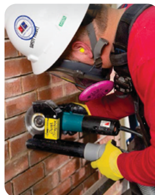
Grinding mortar using dust vacuum device
